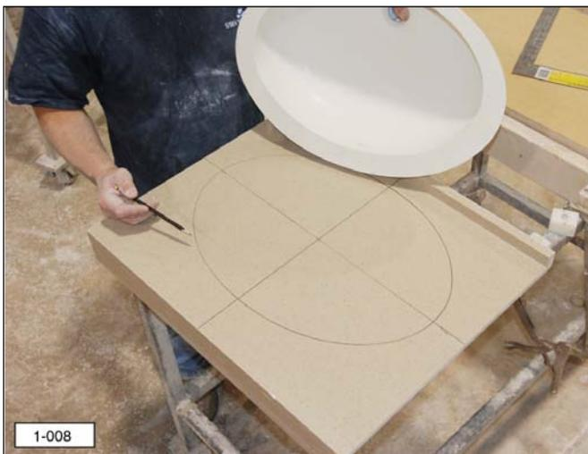
5. Thoroughly sand the underside of the countertop, inside the sink outline, with 36 grit sanding pads. Sand an area 3 inches wide up to the pencil line. Remove all gloss and rough up the surface to allow for proper adhesion. Do not remove the pencil mark of the sink outline.
