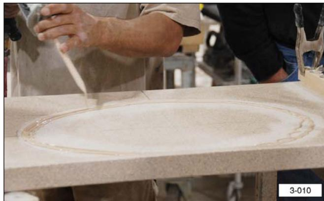
11. Use a spread stick to smooth out the adhesive. The adhesive should be just thick enough to hide the countertop surface underneath.
