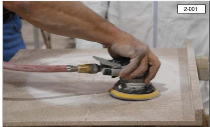
6. Thoroughly sand the rim of the sink with 36 grit sanding pads. Remove all gloss and rough up the surface to allow for proper adhesion.
