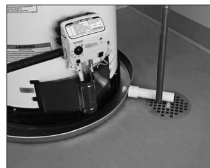
Figure 14. A metal drain pan piped to an adequate drain can help protect flooring from leaks and drips.
