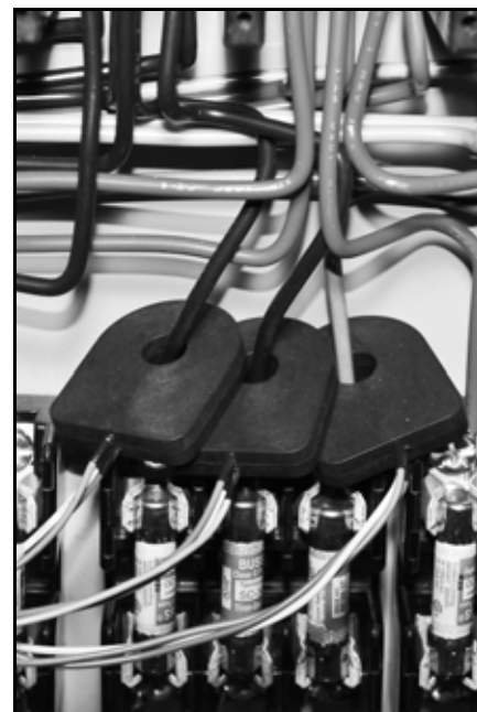
Heating Element Wire Routing
