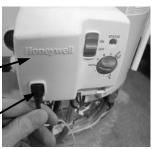
Step 9. Remove the burner assembly from the combustion chamber.
