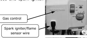
Remove the gas control & thermal well by rotating Step 6. the flats of the Thermal Well counter clockwise using a 1-5/16" wrench. Flats of thermal
