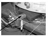
Step 10. Remove manifold mount from burner inner door by removing (2) 1/4" hex drive (2) 1/4" hex drive
