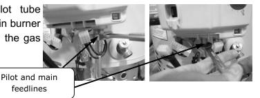
Step 5. Disconnect the wire harnesses and spark igniter/ flame sense wire from the gas control.
