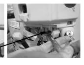
Step 5. Disconnect the wire harnesses and spark igniter/flame sense wire from the gas control.
