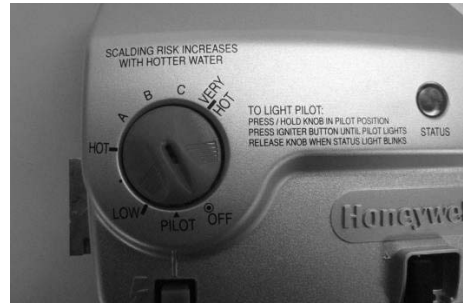
Gas Control shown in the "OFF" position
