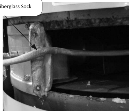
Position Fiberglass Sock
