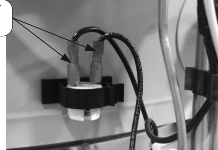
Flammable Vapor Sensor Harness Leads
