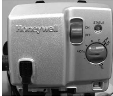
Gas Control shown in the "OFF" Position
