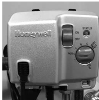
Gas Control shown in the “OFF” position
