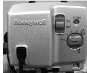
Gas Control shown in the "OFF" Position
