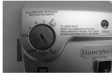
Gas Control shown in the "OFF" position
