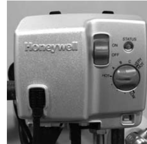
Gas Control shown in the “OFF” position
