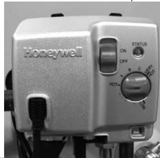
Gas Control shown in the "OFF" position
