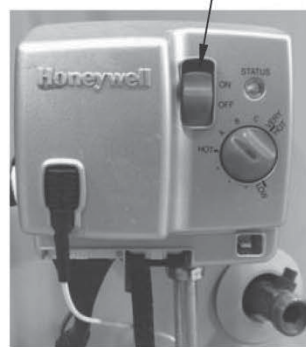
GAS CONTROL SHOWN IN THE "OFF" POSITION
