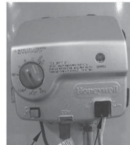
IGNITER WIRE RED AND WHITE PILOT WIRES
